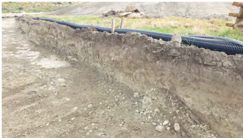
Photo 2. Depth of subgrade cut (0.3 – 1.2m). Illustrating soil profile along Stage 'B' / 'C' boundary
