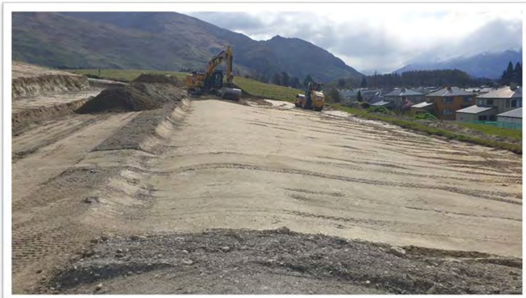
PHOTO 1 - SITE PHOTO OF FIRST 600MM FILL LAYER, LOOKING WEST, PROOF ROLLING OF SUBGRADE IN BACKGROUND AND CUT EARTHWORKS IN TOP LEFT CORNER
