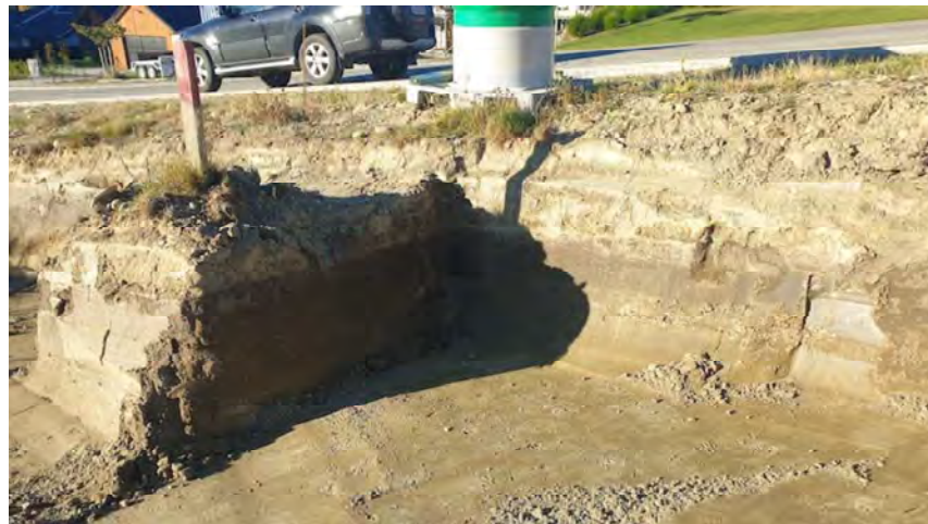
Photo 1. Depth of subgrade cut adjacent West Meadows Drive
