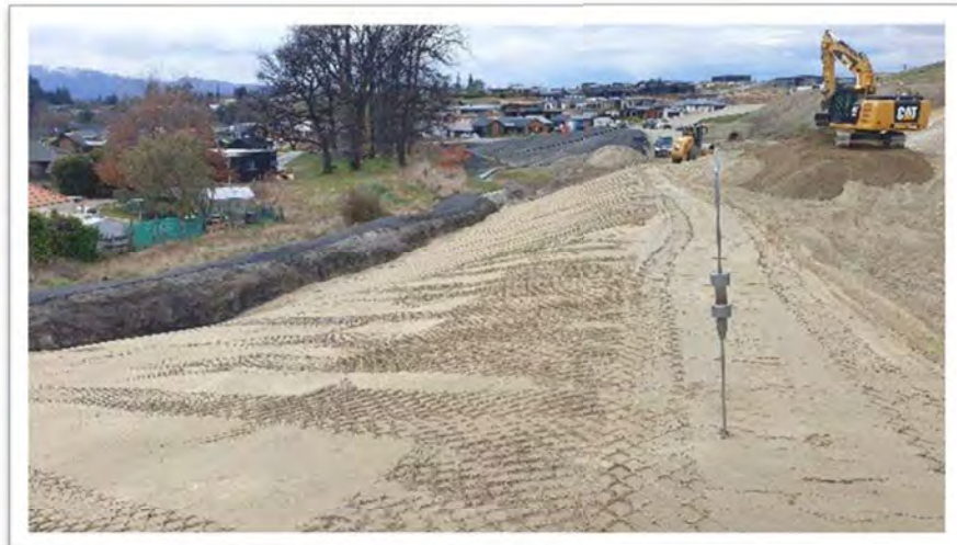
PHOTO 2 - SITE PHOTO LOOKING WEST, ILLUSTRATING -0.6MFL SUBBASE SURFACE, SPT106/GPS833 IN FOREGROUND
