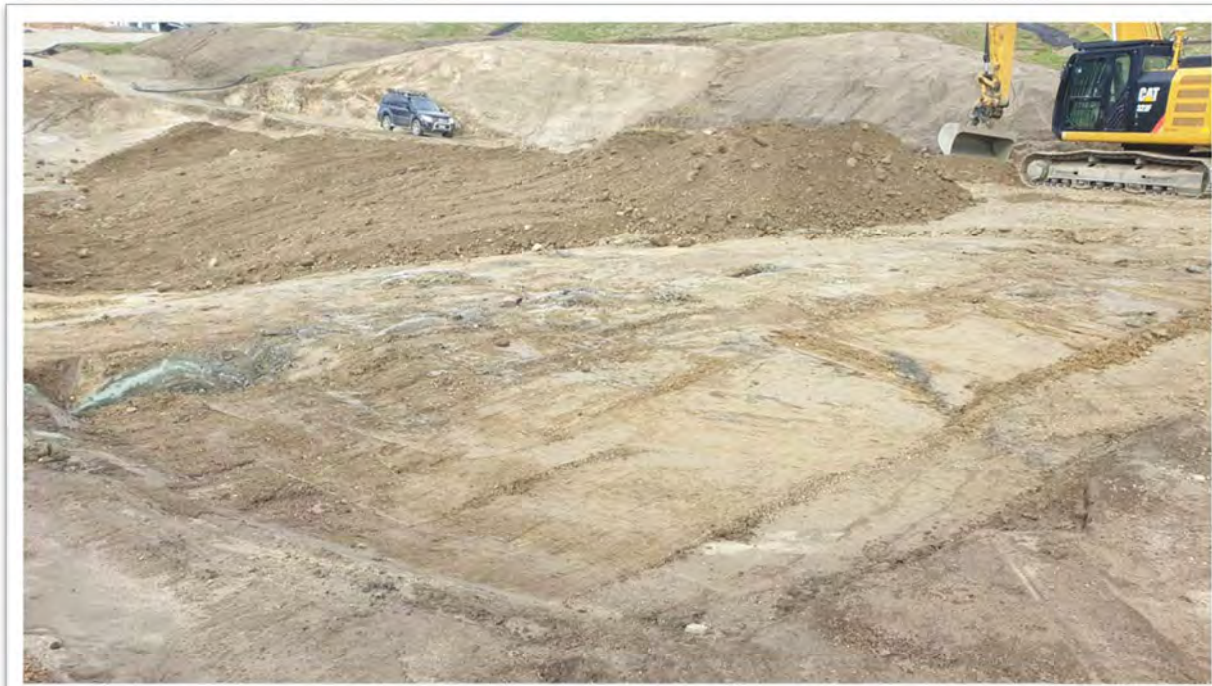
PHOTO 1 - SITE PHOTO LOOKING TOWARDS THE SOUTHEAST, LEFT: (AREA NO. 1) FIRST 600MM FILL CONSTRUCTED (~ 1.8MFL). CENTRE: 300MM LOOSE FILL LAYER OVER MAIN FILL AREA. RIGHT: IMPROVED SUBGRADE SURFACE.
