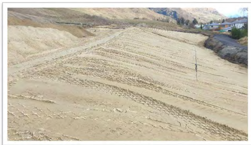
PHOTO 2 - SITE PHOTO LOOKING WEST, ILLUSTRATING -0.6MFL SUBBASE SURFACE, SPT106/GPS833 IN FOREGROUND
