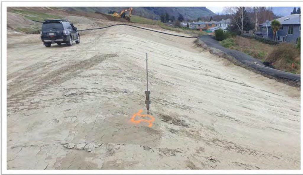
PHOTO 1 - SITE PHOTO LOOKING WEST ILLUSTRATING FINAL GROUND PROFILE, SPT101 /NDM 55 IN FOREGROUND
